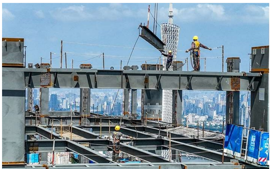
Guangzhou Pazhou Artificial Intelligence and Digital Economy Pilot Zone under construction, Sept. 3rd, 2022. (Source: Visual China Group)
